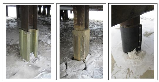
Figure 8. H-Shaped, Rectangular, and Pipe Pile Protective Systems
