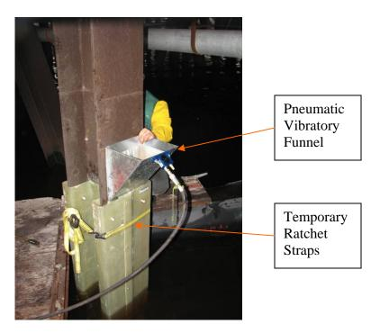
Picture 8: H-Jacket with Ratchet Straps and Vibratory Funnel
