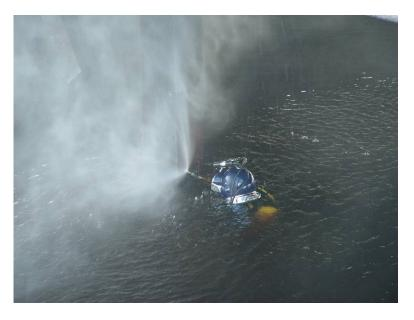
Picture 1: Diver Performing Blast Cleaning
