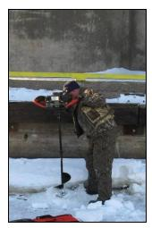
Individual holes were drills for each pipe and anode (ice was ~4 feet deep along pier).
