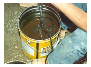
Picture 9: Mixing SeaShield 550 Epoxy Grout
