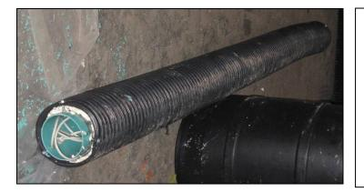
The 6" diameter pipe was then installed in and attached to an 8" corrugated PVC pipe (typically used for culvert installations). The top void between the two was sealed with expanding foam insulation to prevent heat loss from between the two pipes.
