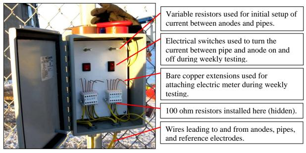
Picture 30: Weatherproof Testing Cabinet Installation
