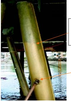
Grout Line Being Pumped Up Jacket
