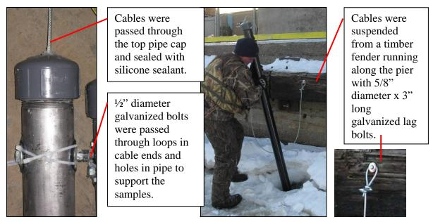
Pictures 18 & 19: Pipe Sample Cable Support Installation
